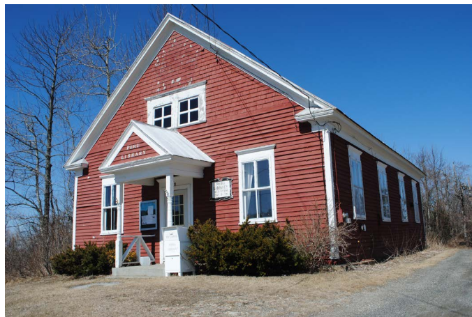
The library in Peru, Massachusetts, received a fiber connection to the MB123 network, which serves important community institutions.
