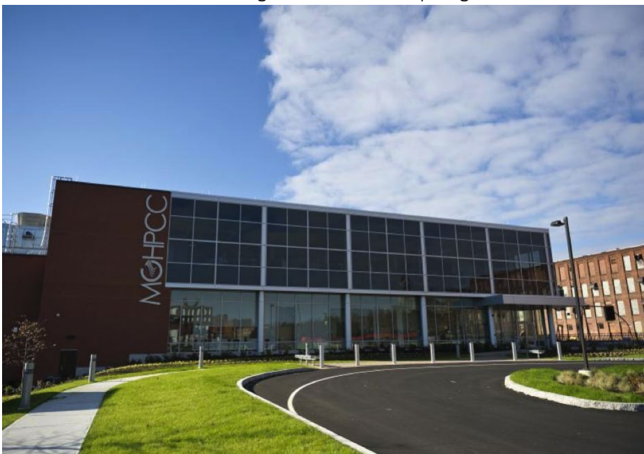
The Massachusetts Green High Performance Computing Center
